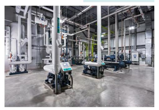
Within the motor room pictured above, there are various colors of piping. The silver coated piping contains ammonia, while the white piping houses CO2, and the green piping is dedicated to glycol.
